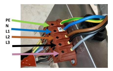
The mains supply connection is made at the rear of the generator. It is desirable that the 5 conductors be fitted with ferrules at their ends.
